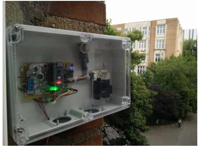
Fig. 2. Board placement during the testing process
